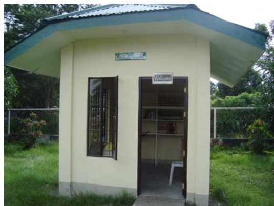
Silway-8 BCPC Building/Reading Center inside the Barangay Hall Compound.
